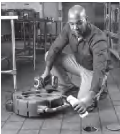
Figure 13 – Applying Lubricant to the Cable Sheath
