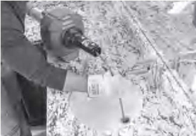
Figure 14 – Manually Feeding Cable
