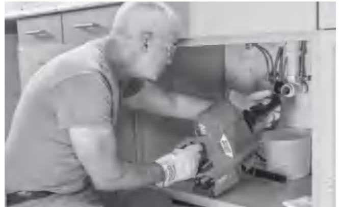
Figure 13 – Feeding Cable With AUTOFEED Unit
